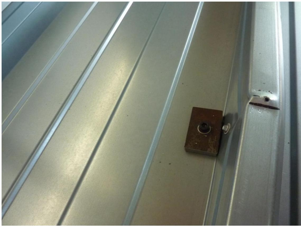
Figure C.7: Screw hole in the middle of the span (IS W-110-075-1242-2 and IS-W-110-100-1242-2)
