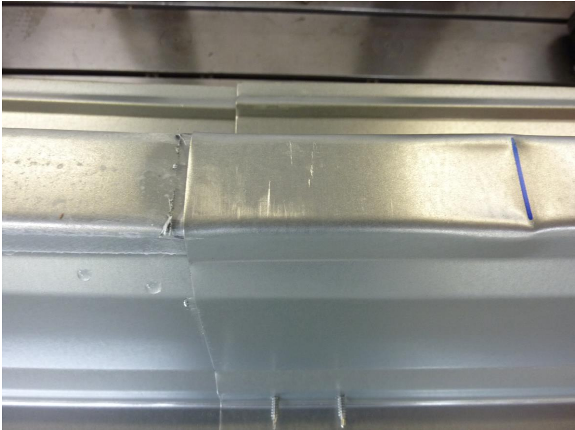
Figure B.12: Failure mode (exemplary IS-135-DIN-160-75-240-1)
